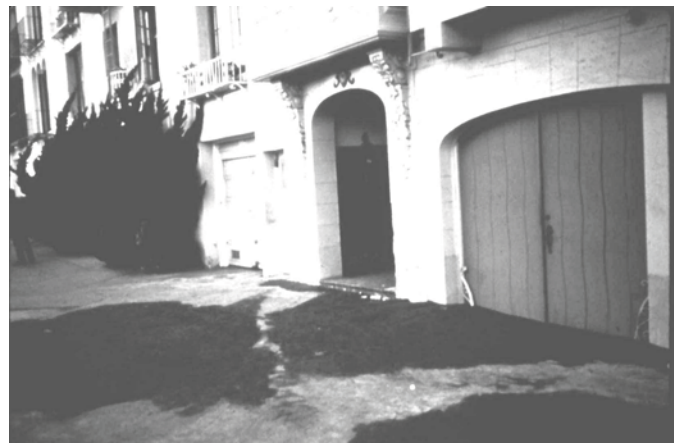
Figure 40 - Loma Prieta Earthquake, October 17, 1989. Lateral spreading, liquefaction and sand boils caused extensive damage in the Marina District of San Francisco, about 60 miles away from the epicenter.
