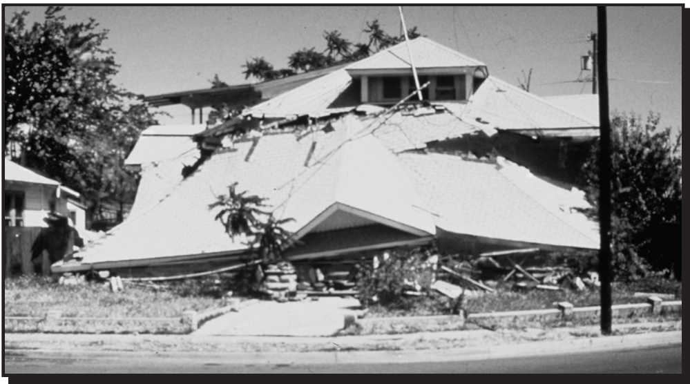
Additional damage from aftershocks
